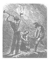
After we have drilled the hole, we clean it out with a scraper and fill it with gunpowder. A lump of clay is used to block up the end of the shothole and a pricker is used to make a hole through the clay for a fuse. Prickers are made of copper or bronze to prevent sparks causing the gunpowder to explode a bit too early. Our fuses are made of hollow straws and in September we go into the fields after the corn is harvested to
