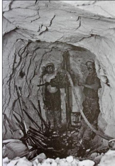
Compressed Air Drilling Machine
